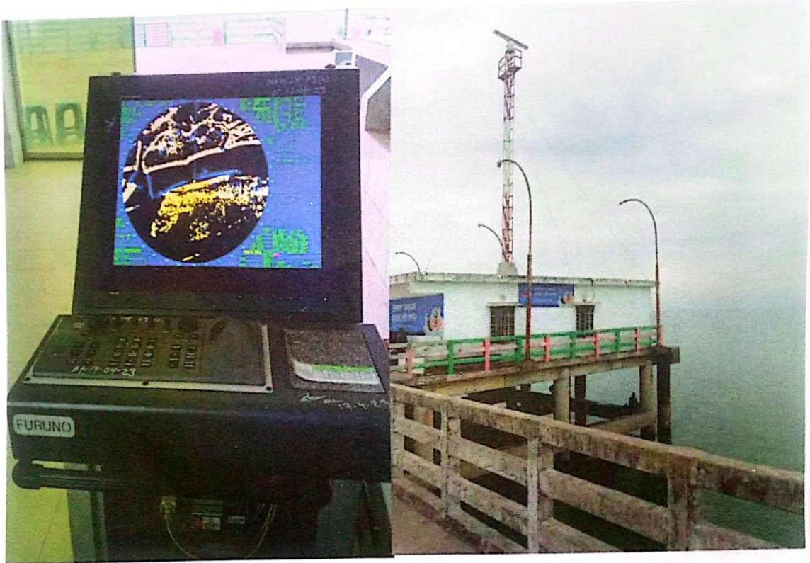
Surveillance RADAR of Teknaf Jetty Ghat
